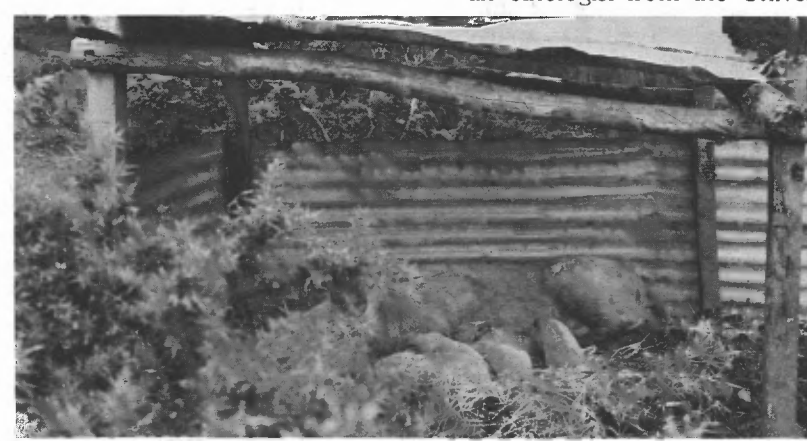
Sows on the hillside built nests for their piglets. Dr. Stolba added the tin roof and walk to the nest site for extra protection.
