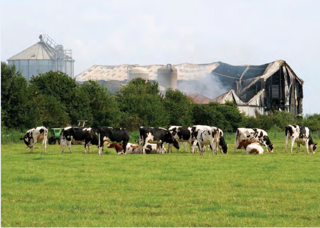
As cows graze on pasture, a fire-destroyed chicken barn smolders in the background.
